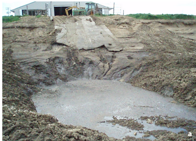
Figure 3. Erosion of an earthen manure storage (source: USDA-NRCS).
