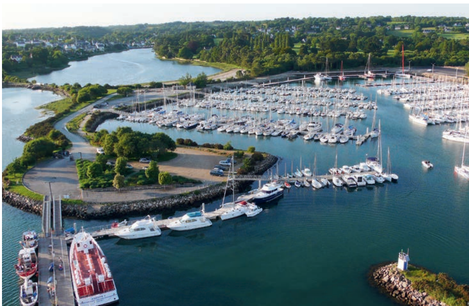
Figure 4. Port-La-Fôret harbour before its much-needed sediment remediation project. A plan conceived by between port authorities, engineering and design departments, France's EPA equivalent and local communities involved pumping 40,000 cubic metres of sediment to a dewatering site located four kilometres inland from the harbour. Photo Ronan Quemere, courtesy of Office de Tourisme de La Forêt Fouesnant
