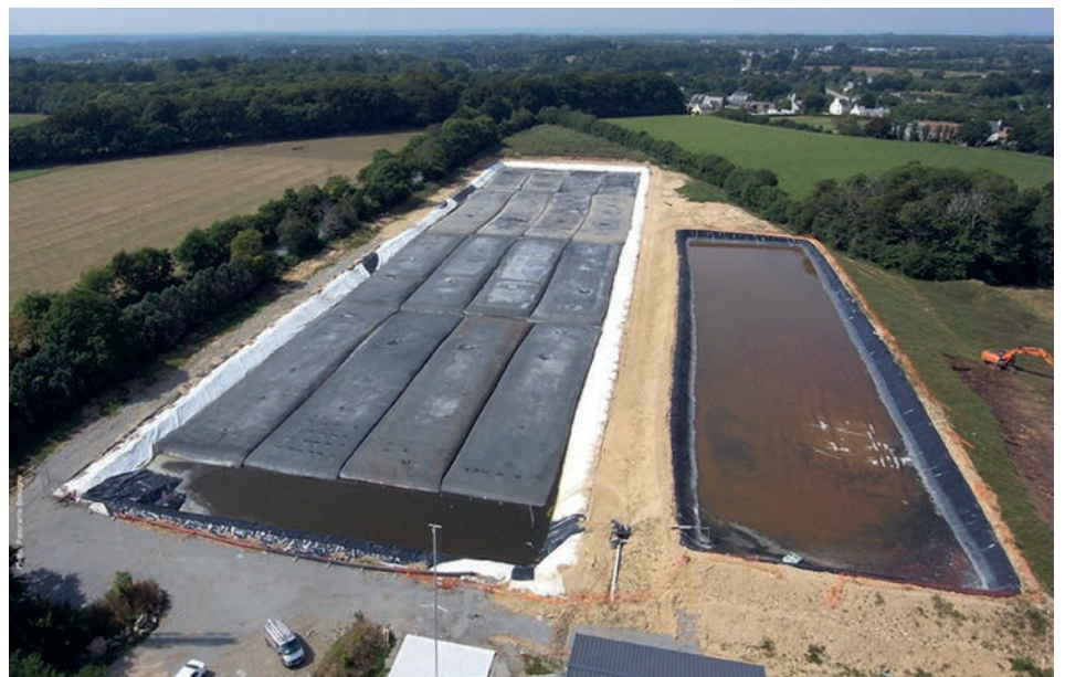
Figure 6. For the project at Port-La-Forêt harbour, the sludge treatment area includes a dewatering area with tubes (left) and water retention area (right).
